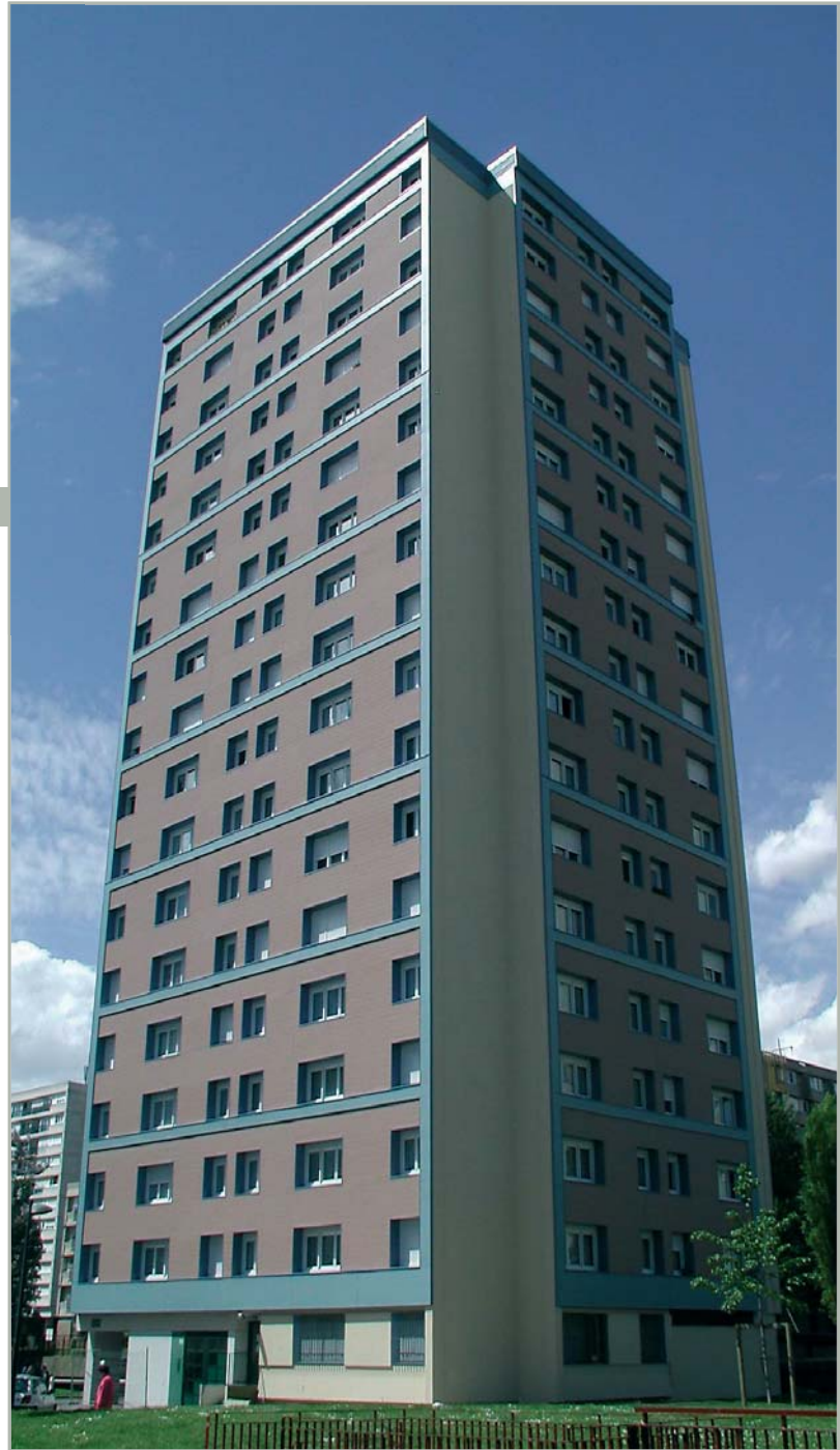
High-rise building in Paris, F
